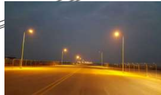
Breaking the darkens in Karbala refinery project roads
